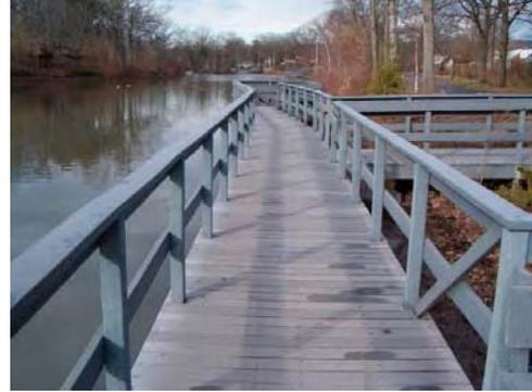
FIGURE 7. COMPOSITE DECKING FROM US PLASTIC LUMBER
